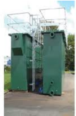
Separator complete with tank and corrugated plate packs.
