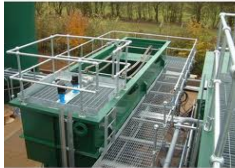
Separator complete with tank and corrugated plate packs.
